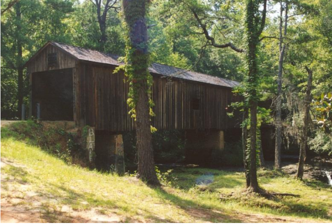
Coheelee Creek Bridge
